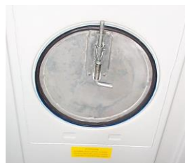
Figure 9.11 Roof hatch internal lock
